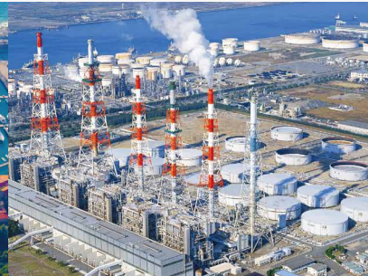
Energy Pipeline Patrol
